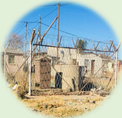
1. Tlhakalatlou Pump station
