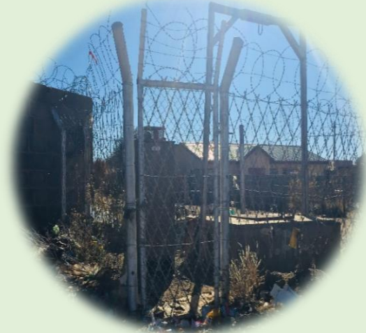
2. Kuilsville Pump station
